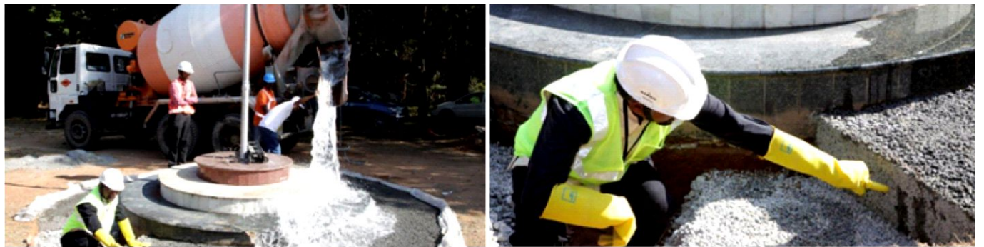
Demo On Pervious Concrete by RMC Ready-mix India Ltd
